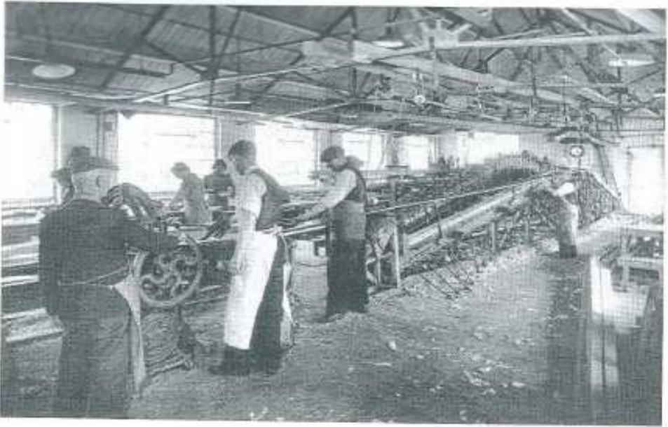
The machine in the foreground looking like an old-fashioned mangle is a hand-driven glue spreader. The rollers rest in a trough of glue, depositing it on the timber as it passes through. In the background are the cramping jigs where the spar booms are built up with these laminations of spruce timber.
